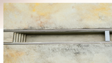
Detail of undertrack inspection pits.
